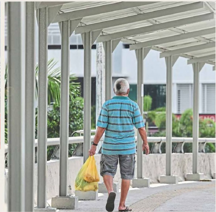
An elderly resident using the newly completed covered walkway.
