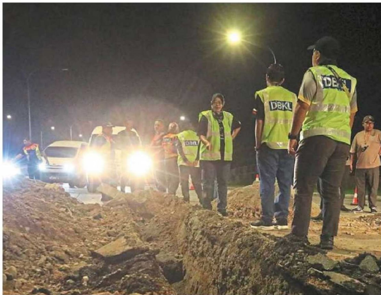
DBKL and CIDB personnel inspecting a road excavation contractor in Kuala Lumpur. — Courtesy photo
