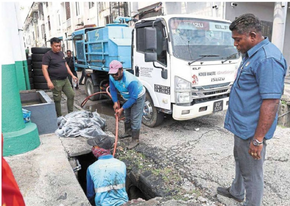
Murugiah (right) monitoring the cleaning of drains by KDEB contractors during the joint operation in TTDI Jaya. — Courtesy photo
