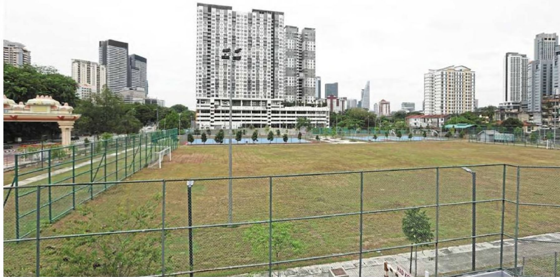
Residents are still unable to utilise the 2.42ha site with a new football field, basketball court and futsal court more than a year after construction has been completed. — YAP CHEE HONG/The Star
