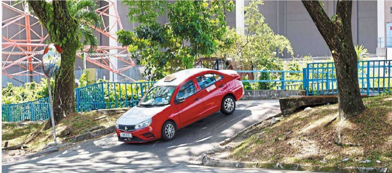
Left: A car using the steep and narrow bridge at Jalan 4/76 in Desa Pandan, which will soon be closed to four-wheelers.
